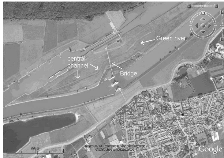
Figure 5.2: Aerial picture showing the Green River at Driel and the bridge that was used to take the flow measurements from (picture: Google Earth).
