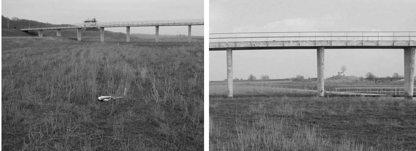
Figure 5.3: The vegetation that covers the channel bed in the Green River at Driel (see Table 5.1 for vegetation characteristics). Below the large bridge that spans the entire Green River at Driel, a small bridge crosses the central deeper channel, as seen in the right picture (pictures by Menno Straatsma).
